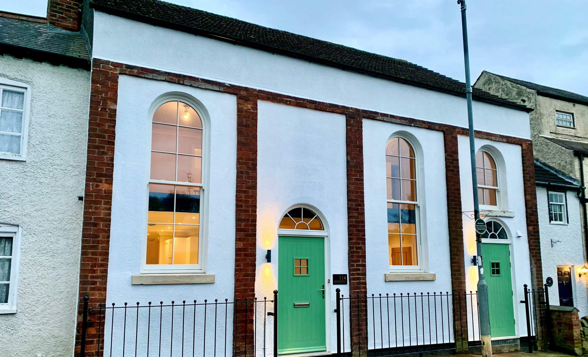
The Former Chapel Main Street Markfield LE67 9UX
